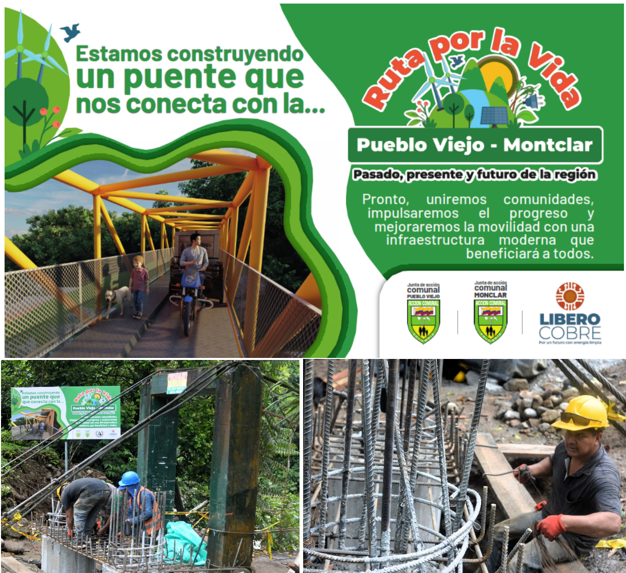
Figure 7 – New Montclar walking bridge under construction.
